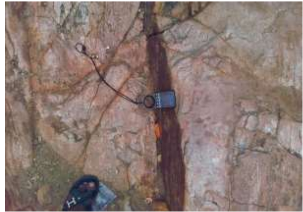
Plate XII: A Dip Slip fault at Angwan Dahariya (N8°59'04" E8°13'55")
