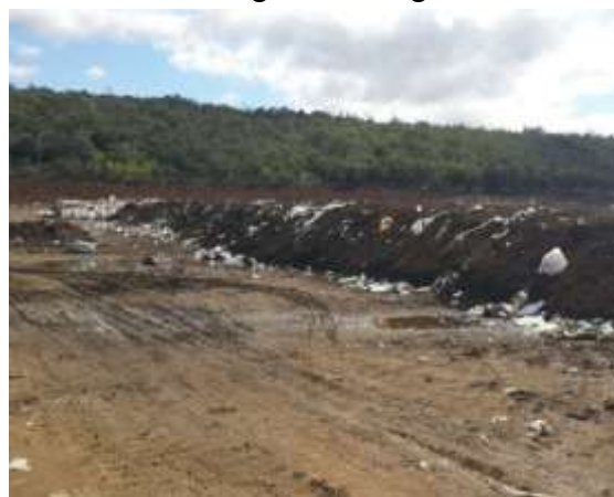
Figure 1b: Dumpsite surface composition viewed from the East
