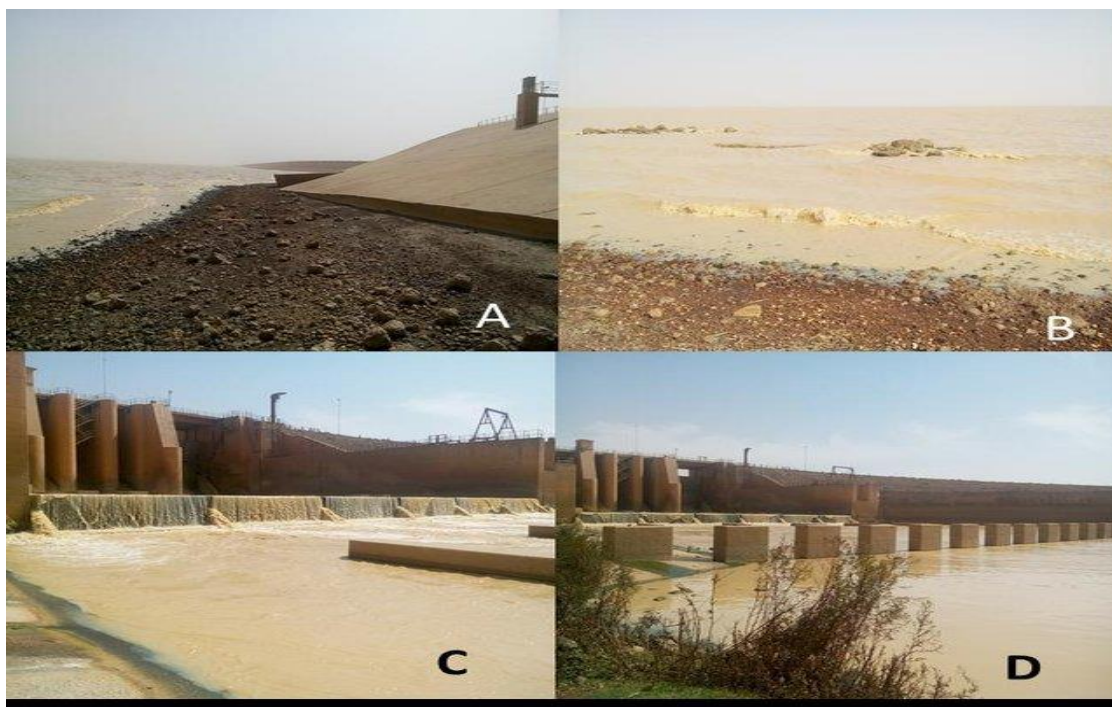
Plate 2. Goronyo Dam Showing Upstream (A-B) and Downstream (C-D)
