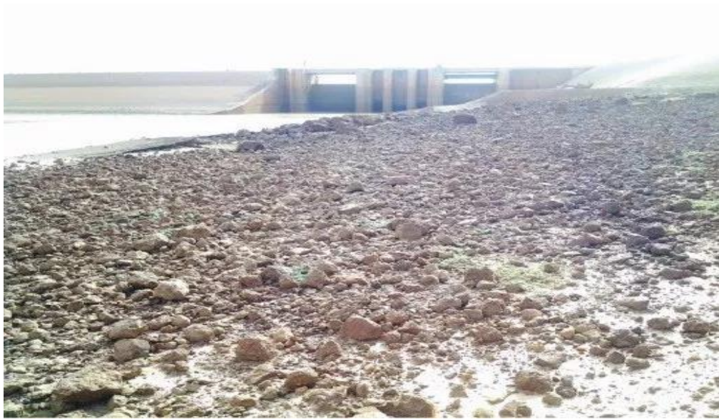
Plate 4. Sand Dome presence in Goronyo Dam
