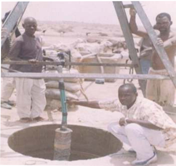
Plate 2: A borehole at Masu drilled into Middle aquifer. Note: The borehole is now turned into hand-dug well with hope of tapping the lowered water level at a greater depth below the subsurface
