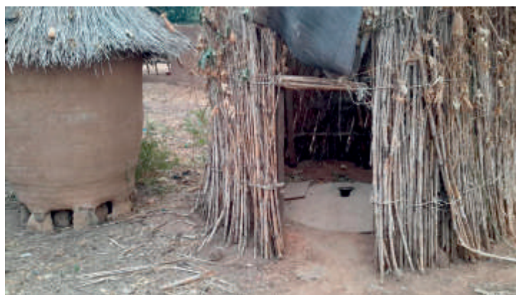
Plate 4. Basic latrine using simple materials at the community level (Gidan Kwano)
