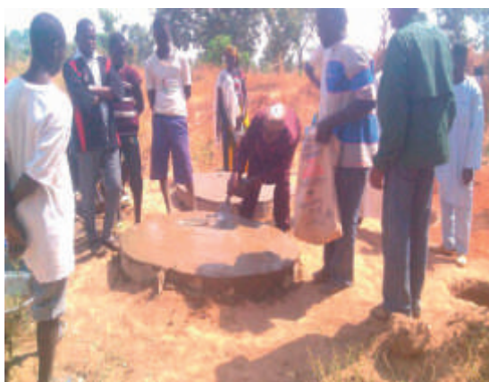
Plate 3. Preparing sanitary platforms for toilets at Garatu area
