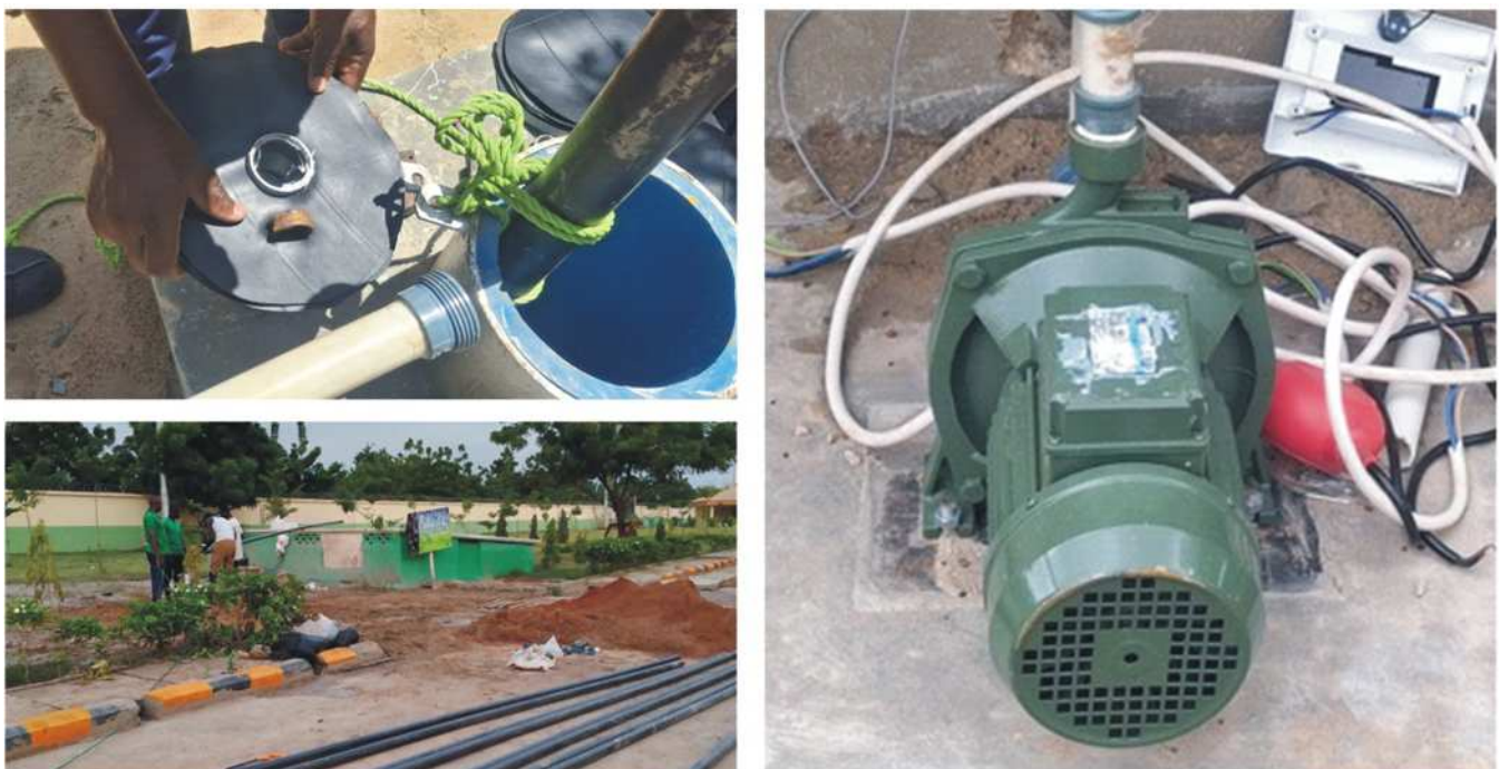
Plate 3: Riser pipes, well top seal and pressure pump used for the installation
