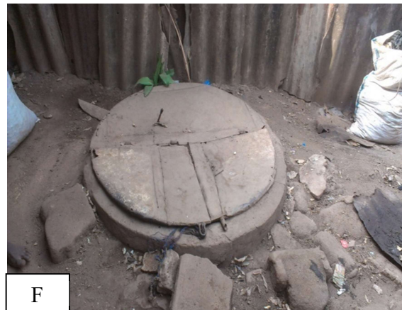
Plate 5: Poorly sited and constructed hand-dug wells in Presco. (A and B are located close to public gutter). (C and F are constructed the same height with ground level). (D and E located at unhygienic environment).
