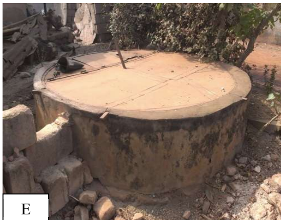
Plate 5: Poorly sited and constructed hand-dug wells in Presco. (A and B are located close to public gutter). (C and F are constructed the same height with ground level). (D and E located at unhygienic environment).
