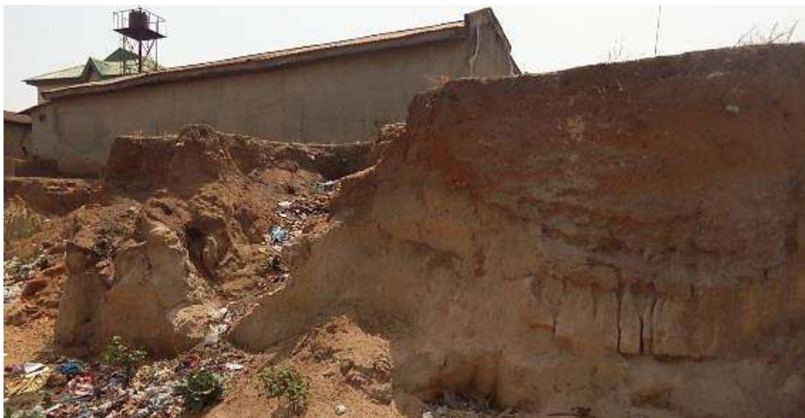
Plate 2: Gully erosion site at Gbongbofu area of Bida Town, Niger State
