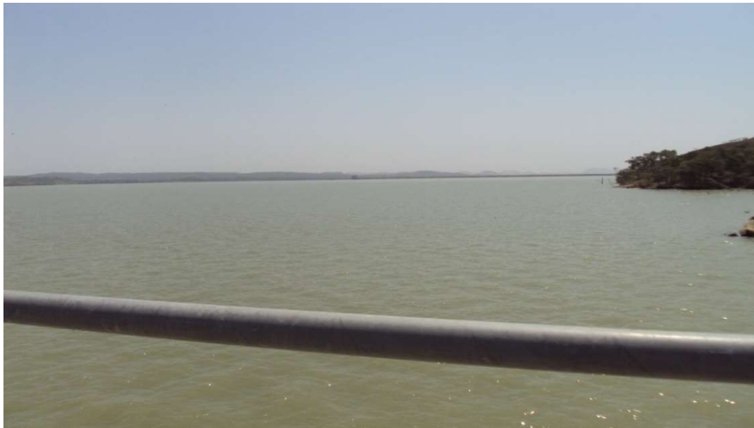
Plate 1. Section of Goronyo Dam from the northern side before 2017
