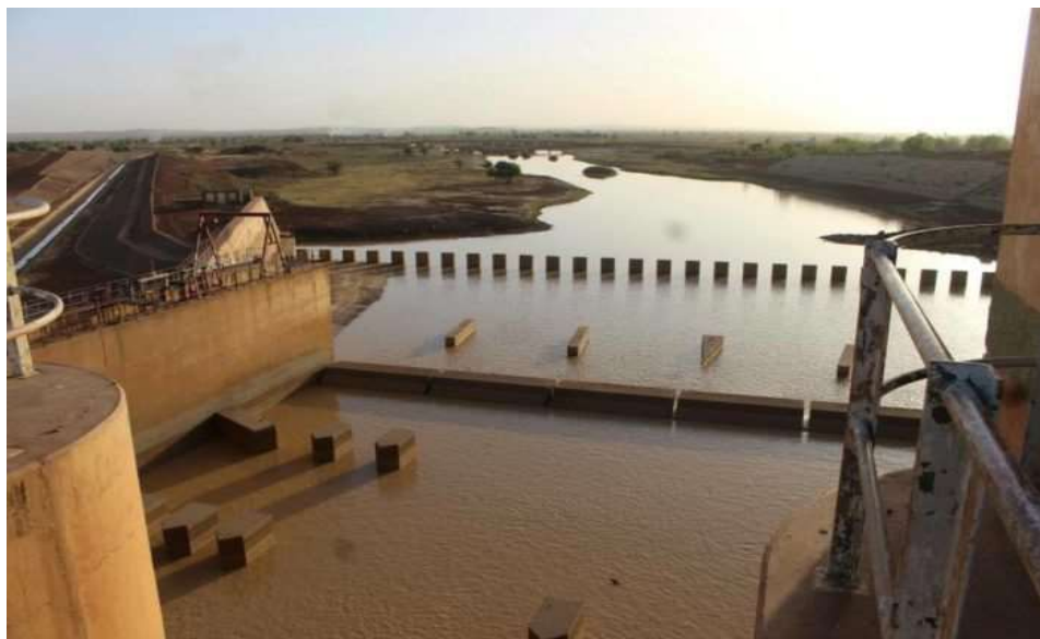
Plate 3. Goronyo Dam water shrinkage from spillway in 2017
