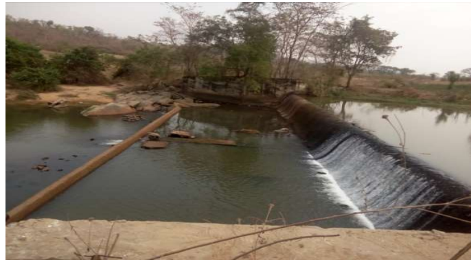
Figure 2: Constructed Oke-oyi dam which is about 1-3 kilometre to study area.
